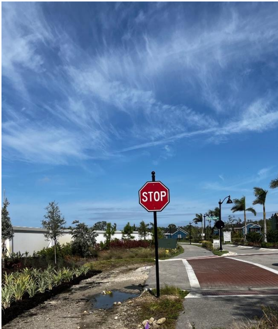
Located near the cove at west port stop sign is facing opposite direction.
